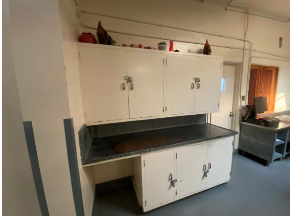
White painted cabinet components contain lead-based paint
