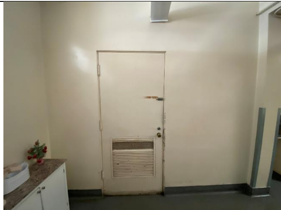
White painted wood door components on the north side entrance of the kitchen contain lead-based paint
