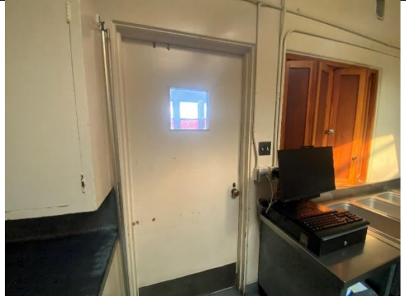
White painted wood door components in the kitchen contain lead-based paint
