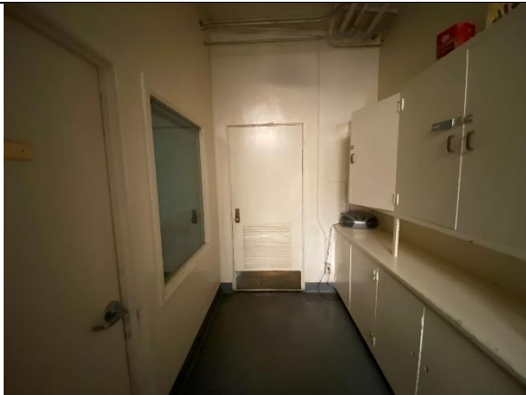
White painted wood door components on the south entrance of the kitchen contain lead-based paint
