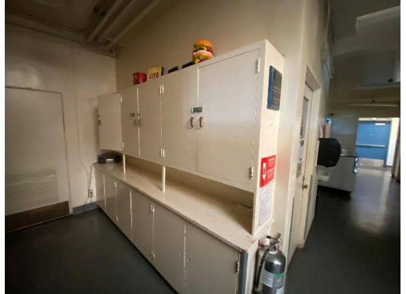
White painted wood cabinet components contain lead-based paint
