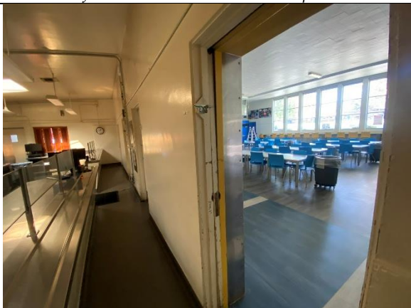
All white/yellow painted wood door components on the shared wall between the kitchen and cafeteria contain lead-based paint
