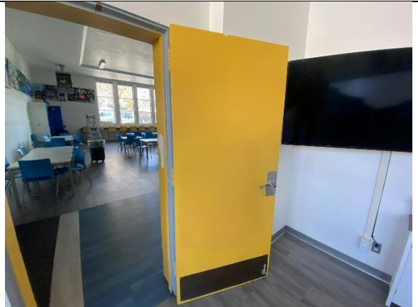
Gray/yellow painted wood door components in the staff lounge contain lead-based paint
