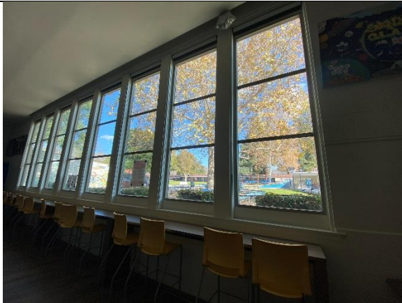
White painted wood window components in the cafeteria contain lead-based paint
